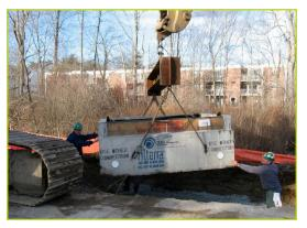
Two 10' x 6' and four 8' x 6' standard Filterra units were installed along Shea Boulevard to treat stormwater runoff. Native plants such as Serviceberry were installed to complement the existing landscape along the street.
